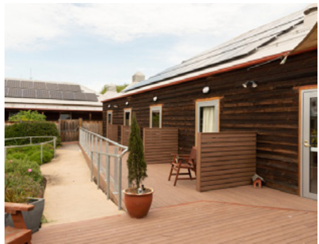
The introduction of doors to the resident rooms allows direct access to the deck and courtyard.
