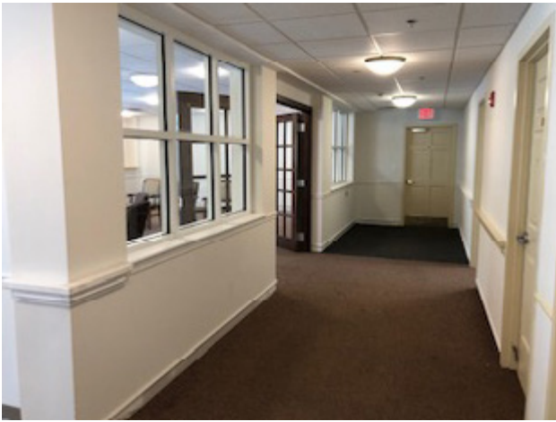
There is an Activity Space at the end of a corridor, minimizing the visual attractiveness of the exit door beyond.
