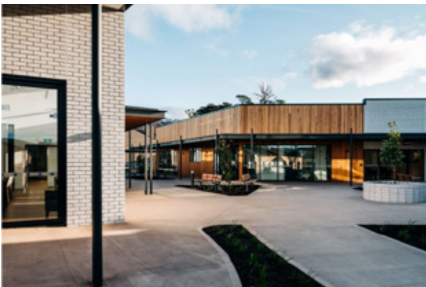
The village design, which features 12 houses in 4 cul-de-sacs, a community centre, salon, a general store, café and wellness centre. It has been informed by extensive research on best practice models of dementia care.
