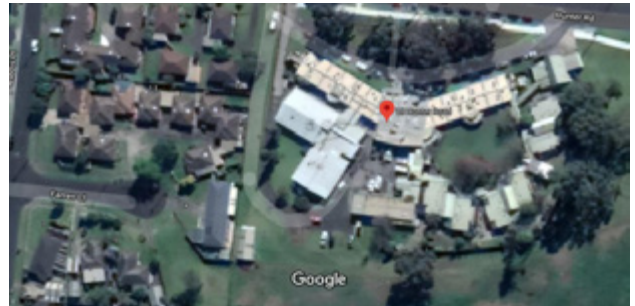
Aerial view of the 3 x 8 bed cottages around a central secure garden and showing the secure rear gardens. Chapel is in a separate building in garden setting. The whole external perimeter was planted with River Red Gums to provide a landscape back drop.
