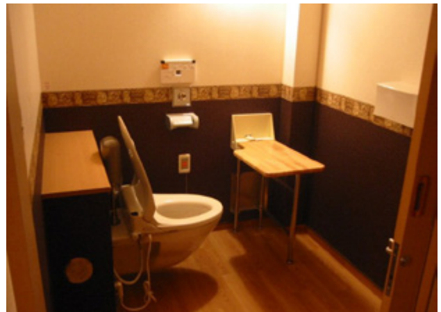
Toilet with flip up table: The table helps the elderly to stand up and sit down, and provides a stable sitting position. In addition, it provides more comfortable posture for using the toilet with ease.
